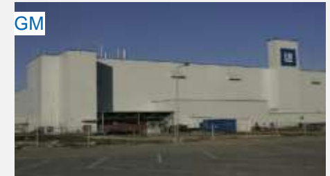
GM Poling & road infrastructure construction
